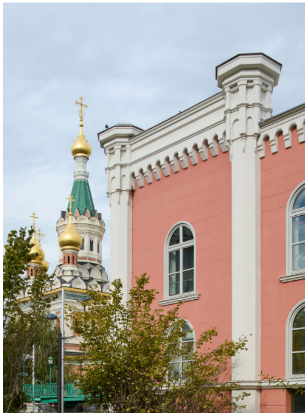
BWM Imperial Riding School/ facade church © BWM Designers & Architects / Lukas Schaller
