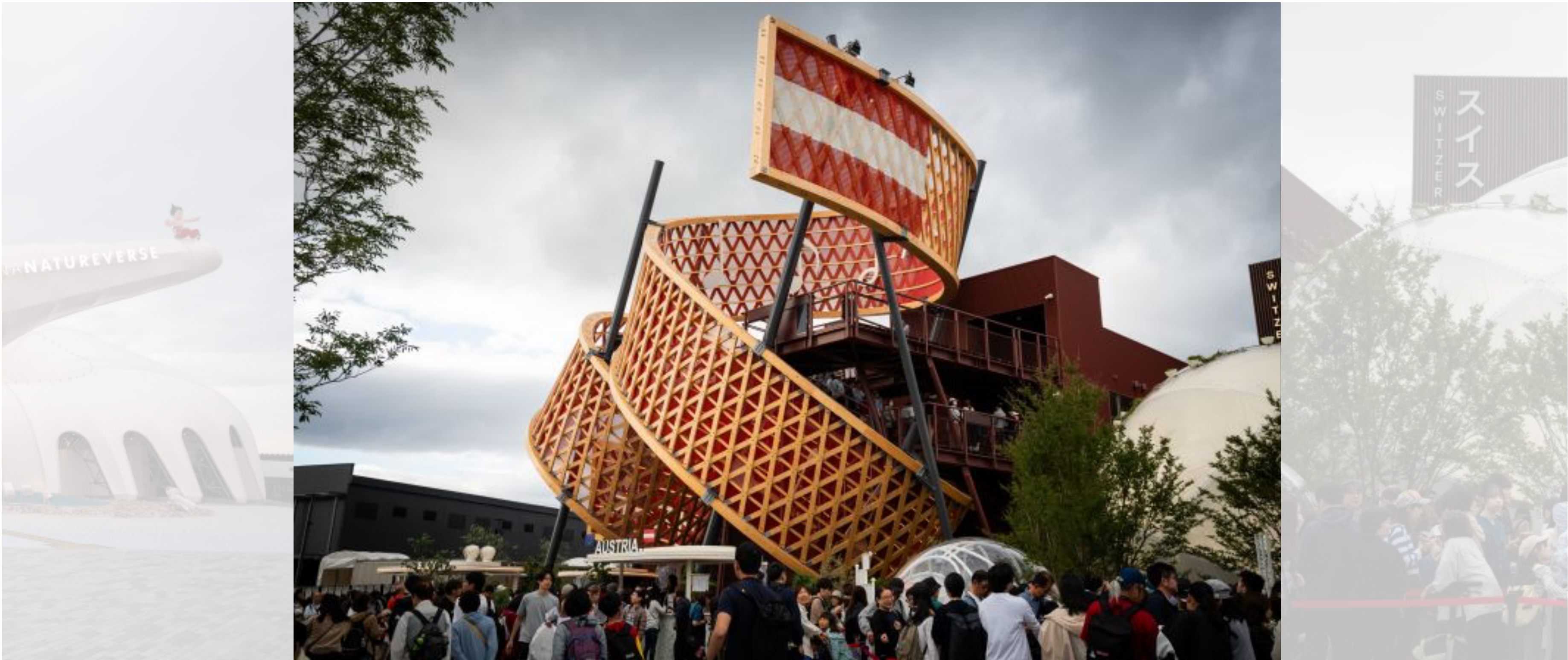
8 of 20 On the theme of “composing the future,” the Austria Pavilion features a distinctive wooden spiral: a 91-meter-long, 4.3-meter-wide ribbon which represents a giant musical score, and includes the opening bars of Beethoven’s Ode to Joy. According to the pavilion’s architects , the wooden structure showcases Austria and Japan’s shared timber craftsmanship while minimizing carbon emissions. Yumi Asada/CNN
